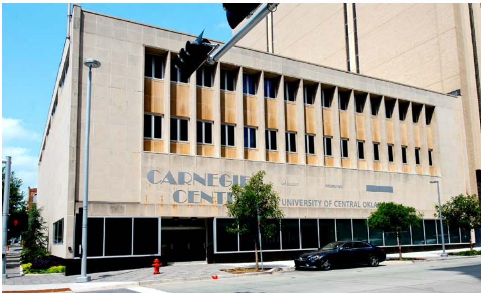
Figure 2. Carnegie Center, home of the UCO Downtown teaching facility
