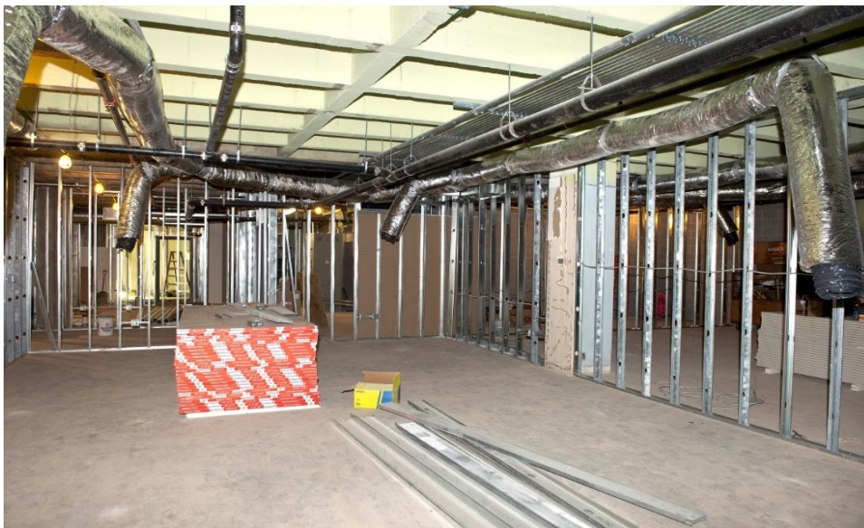
Figure 4. Construction as the HVAC goes in
