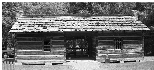
Figure 1.—Grayson dogtrot south façade. Dogtrot houses have two rectangular rooms and a central hall, all under a continuous roof. The open hall is known as a trot.
