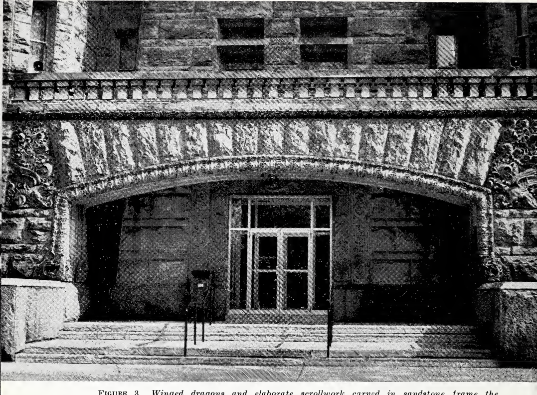
FIGURE 3. Winged dragons and elaborate scrollwork carved in sandstone frame the main entry to the Wood County Courthouse at Bowling Green, Ohio.
