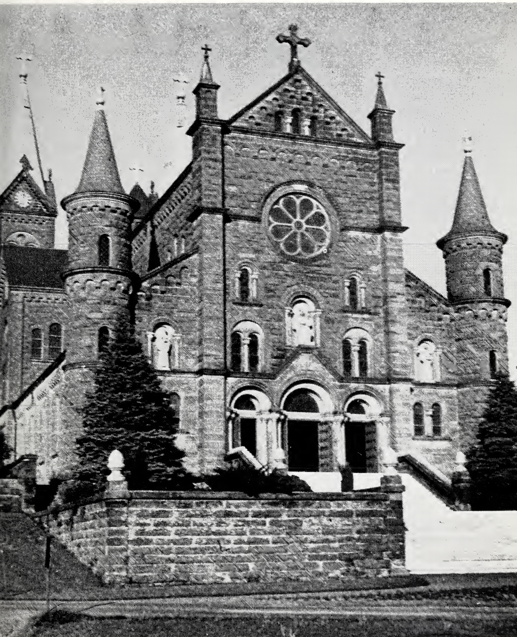
FIGURE 2. St. Meinrad Archabbey in Spencer County illustrates nineteenth-century sandstone masonry at its best. Sand is also a principal constituent of the mortar and the chief ingredient of the stained-glass and other windows.
