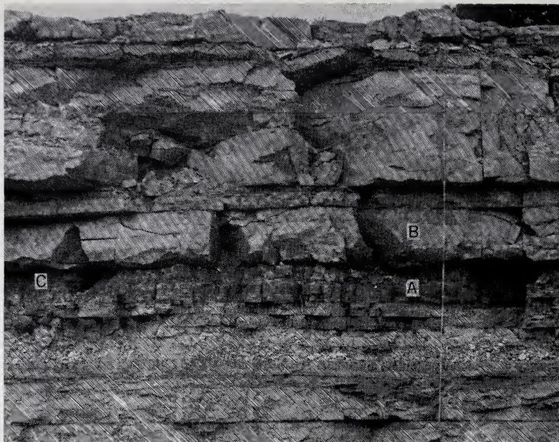
FIGURE 6. Rock cut on west side of new State Highway 37, just south of Gulletts Creek, Lawrence County, showing differences in joint spacing and development of solution channels. Bed A, 1.5 m thick, has joints averaging .25 m apart, whereas joints in bed B, which is about 1.5 m thick, average 2.3 m apart. A filled solution channel at C has developed in the closely jointed bed. Rod is marked in feet.
