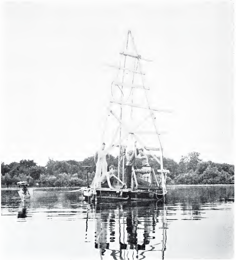
FIG. 1. The float from which drilling in water was done. The force pump is shown in the foreground at the left; the casing between the two middle figures; the tubing, with rubber hose attached, between the arms of the derrick. A block-and-tackle is shown suspended from the derrick and attached to the tubing, and a length of tubing, not in use, is shown projecting above the derrick.
