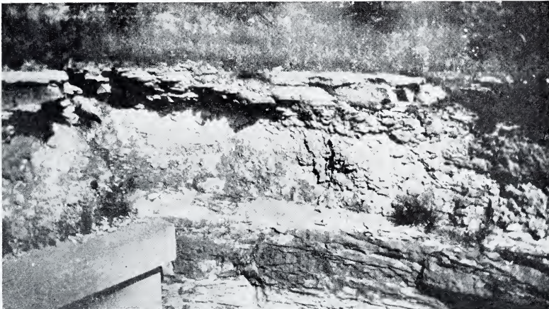
Fig. 2. Contact of the Harrodsburg and Borden at the west end of the Illinois Central railroad tunnel. The limestone is underlain by the basal chert and geode layer. The top of the Borden (Edwardsville formation) is at the level of the top of the concrete.
