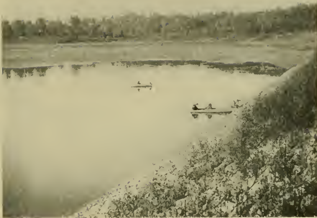
Showing east side of City Waterworks Reservoir, Bloomington. The water is supplied by springs from the underground drainage of sink-hole region in Mitchell limestone.
