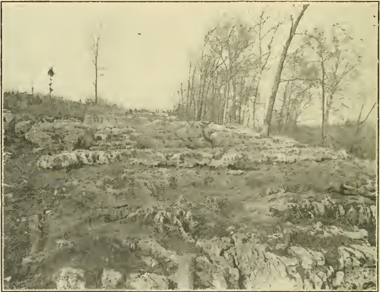
No. 18. Corroded surface of Salem limestone. Oliver Quarry, Clear Creek.
