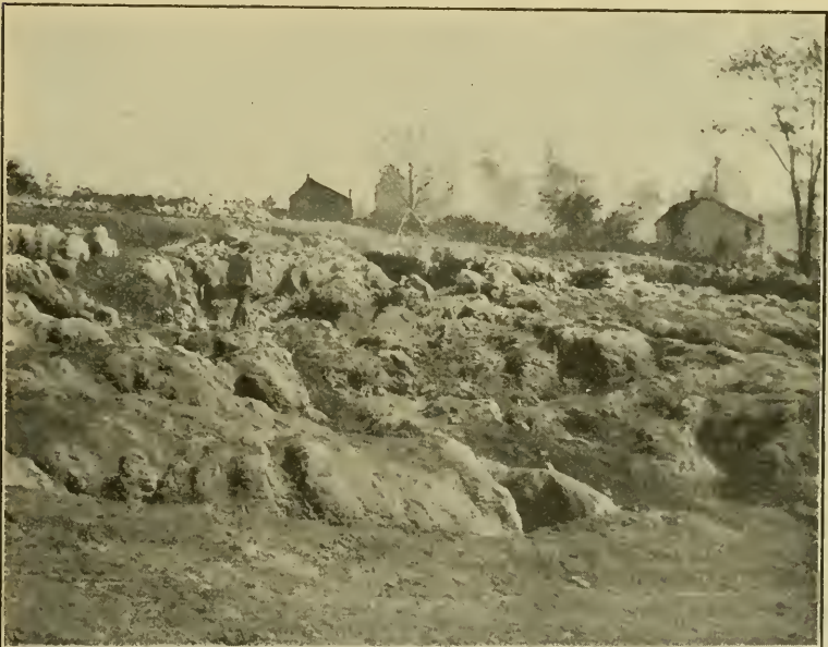
No 20. Corroded surface of Salem limestone. Quarry near Sanders, Ind.
