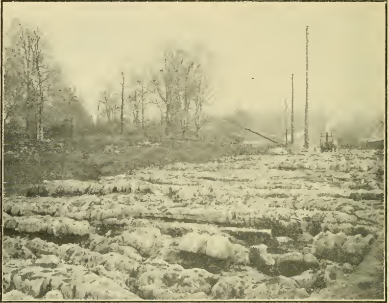
No. 17. Corroded surface of Salem limestone. Quarry near Stinesville.
