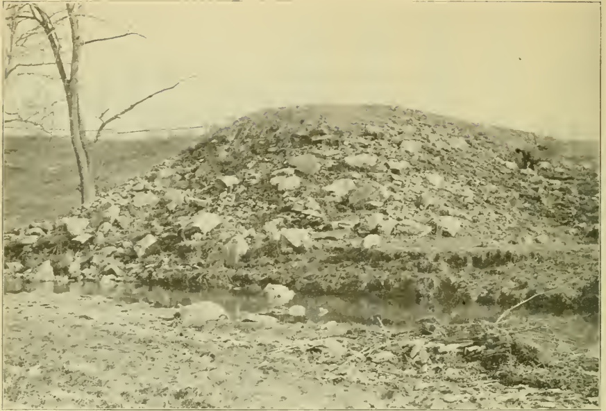
Fig. 3. R. R. fill from material blasted out of cut.
