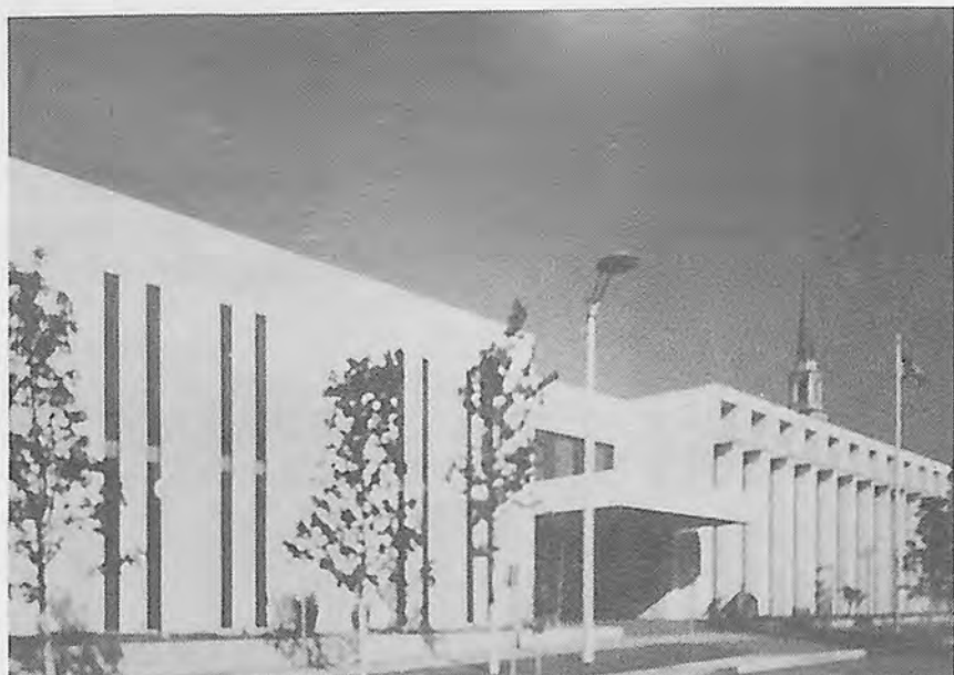
Main entrance, Fort Wayne Public Library, 900 Webster Street, 1970. Photo courtesy of Allen County Public Library.
