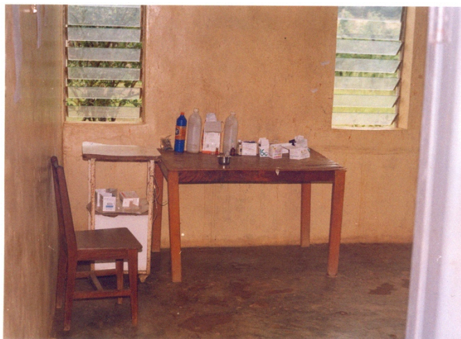
Picture 2. Injection room before renovation
